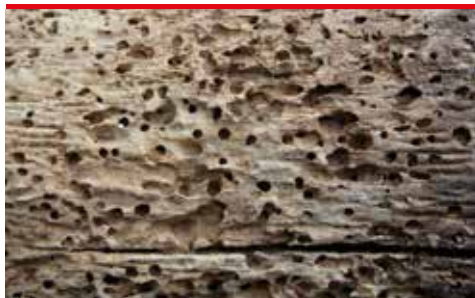
inn 19 Eikeborebille - flyvehull i gml. bjelke (foto - Protox)
