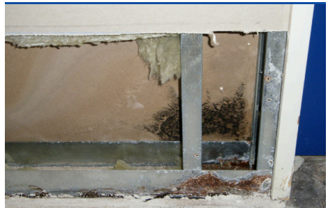
Mould growth ( Stachybotris chartarum ) in light plaster wall after flooding. (Photo: Protox)
