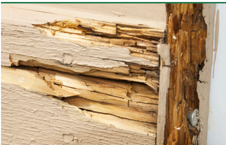
Gilled polypore - degradation in wooden clad- ding in holiday homes. Attack 3-4 years old. (Photo: Protox)
