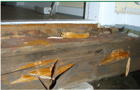
svn 41 Bark fungus – Star hair Bark fungus on wood in basement. (Photo: Protox/Goritas)
