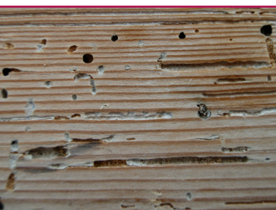
i 11 Common furniture beetles – floorboard with exposed larva passages as a result of planing. (Photo: Protox)
