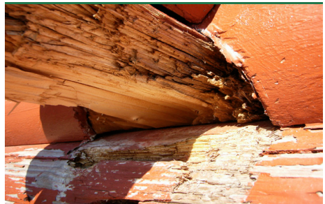
Gilled polypore - decomposition in a log house. (Photo: Protox)
