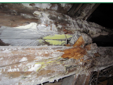
Mine fungus – fruiting bodies and surface mycelium. (Photo: Bøgh & Helstrup)
