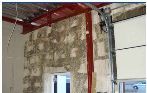
Mould growth on a newly built wall in an industrial hall as a result of construction moisture. (Photo: Protox)
