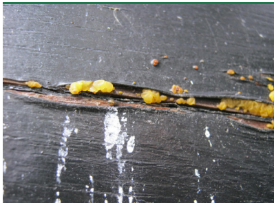
Common jelly spot fungus – fruiting bodies on exterior woodwork. (Photo: Goritas)
