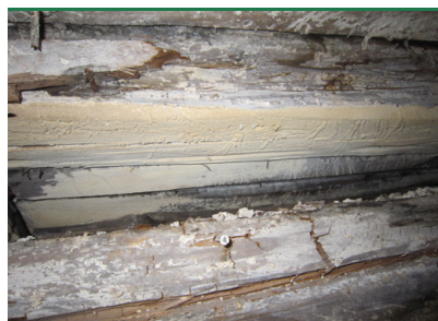
Mine fungus – fruiting bodies, surface mycelium and crevice blocks in floor joists. (Photo: Bøgh & Helstrup)
