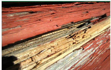
Gilled polypore - leaf decomposition in log house. (Photo: Protox)
