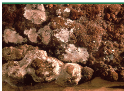
Gilled polypore - sterile fruiting bodies/brown surface mycelium developed in darkness in flat roof. (Photo: Protox/Gori)
