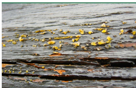
Common jelly spot fungus - fruiting bodies on painted, outdoor woodwork. (Photo: Goritas)
