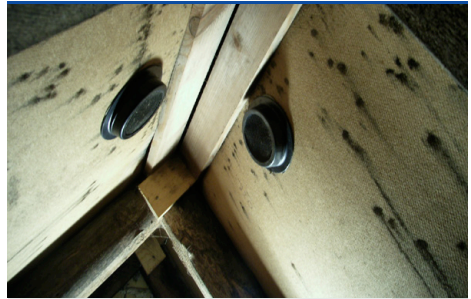
Black mould on the roof due to lack of ventilation of the roof space (valves retrofitted). (Photo: Protox)
