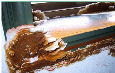
svn 2 Dry rot fungus - fruiting body in window sill of summer house. (Photo: Protox)
