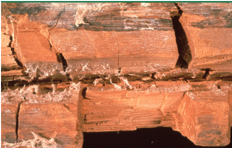
svn 49 Dry rot fungus - broken down wooden beam. Brown rot with large fissure blocks and surface mycelium. (Photo: Protox/Gori)
